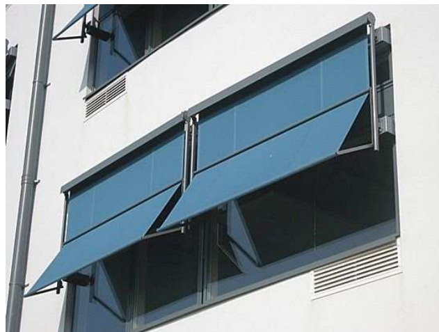
Fig. 53: Example of sunshades on windows to limit the cooling in summer.
