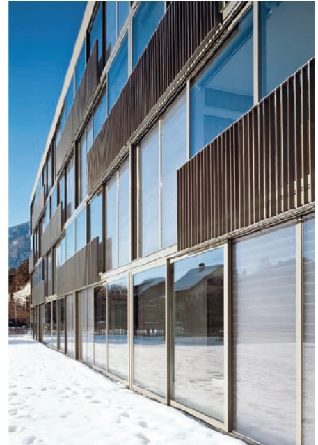
Fig. 53 Close view of the south facade of the senior citizens' apartments with latent heat storing glass facade
