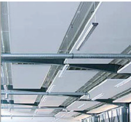
Fig. 40 Installation of ILKATHERM PCM board
