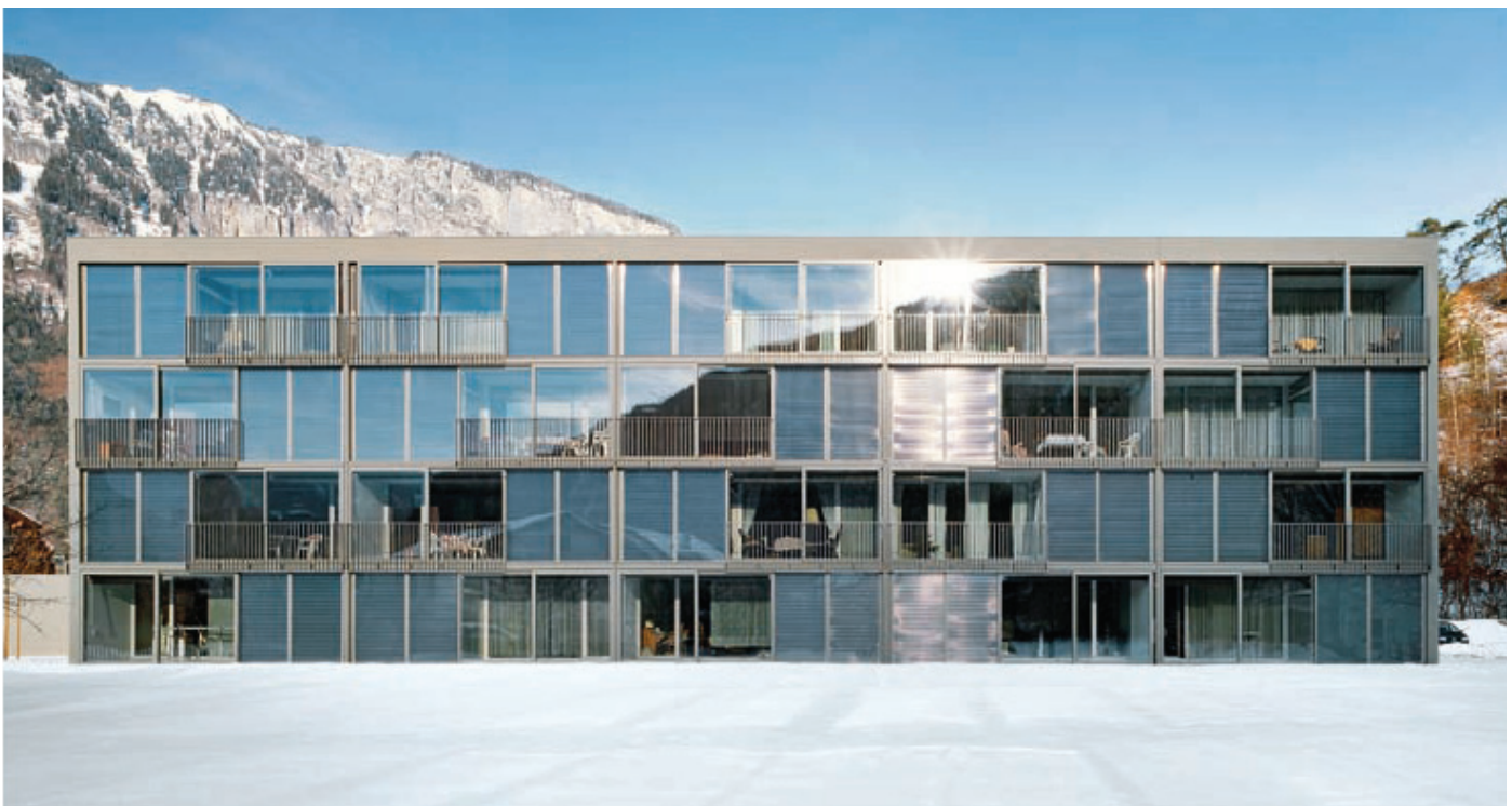
Fig. 54 South facade of the senior citizens' apartments with a latent heat storing glass facade
