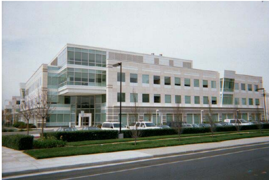
Figure 100. Site #1 – Office Building in San Jose
