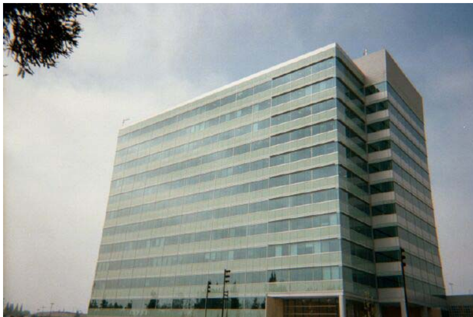
Figure 103. Site #2 – Speculative Office Building in San Jose, CA
