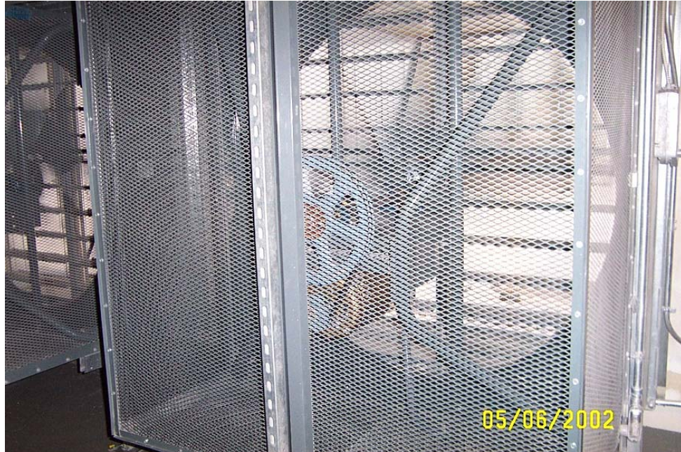
Figure 104. Relief Fan (one of six per penthouse)
