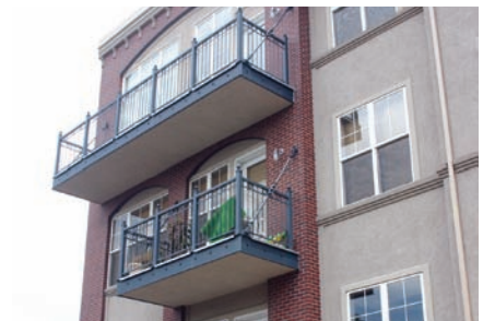
Photo 10: Hang in There. Offset point supports combined with tie rods.
