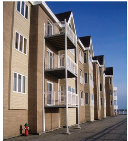
Photo 11: Stand-Alone Balcony. Balconies have their own structural frame and foundation.
