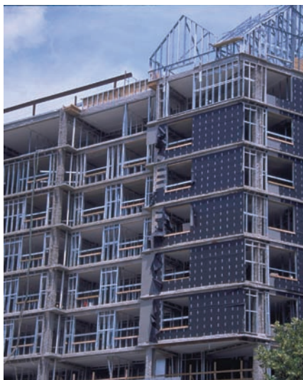
Photo 1 (left): “Harley Davidson” Architecture. The projecting concrete slabs transfer heat across the enclosure. Photo 2 (right): Architectural Statement. Apparently, the projecting slab is visually appealing (who knew?). It catches rain and transfers heat efficiently while wasting floor area (square footage).
