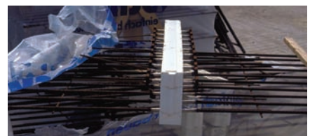
Photo 12: Structural Innovation. Thermal break at slab-balcony connection. Stainless steel rods are welded to reinforcing bars cast into the structural slab. The rods pass through a foam block that acts as a thermal break. The rods are staggered up and down to handle both compression and tension loads.
