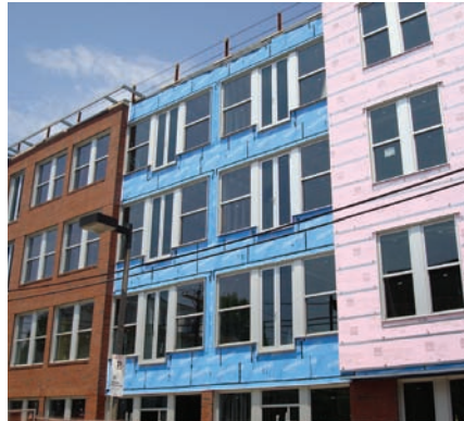
Photo 5 (above): Exterior Insulation. The pink is the exterior insulation. The blue is the rain control layer (drainage plane) and the air control layer (air barrier) and the vapor control layer. The brown is the brick cladding.
