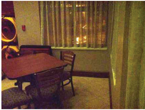
Figure F17. Window sill in a commercial facility.
